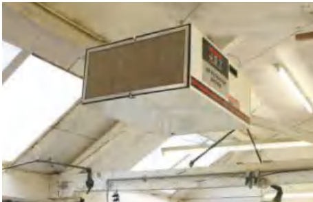
▲ Pic.11 Skylight windows and fluorescent tubes at right angles will ensure you are never working in shadows while a filtration unit extracts airborne dust
